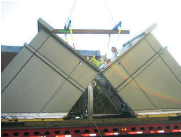
Figure 15: Custom hinged rigging enables units to be shipped flat
