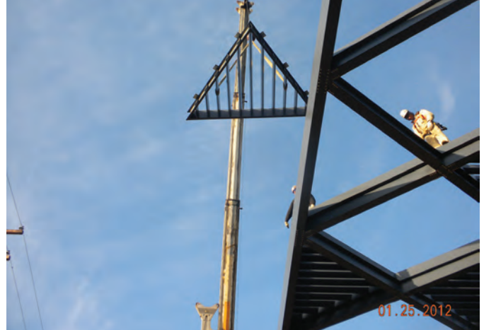
Figure 5: Large triangular shaped sunshade assembly is hoisted into place.
