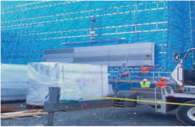
Figure 3: Metalwërks crated wall panels - properly stored awaiting installation
