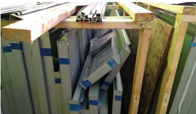
Figure 4: Improper handling of a finished panel. Never leave panel faces unprotected in storage.
